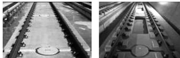
Photo 4 Flat slab (left) and frame-shape slab (right)
