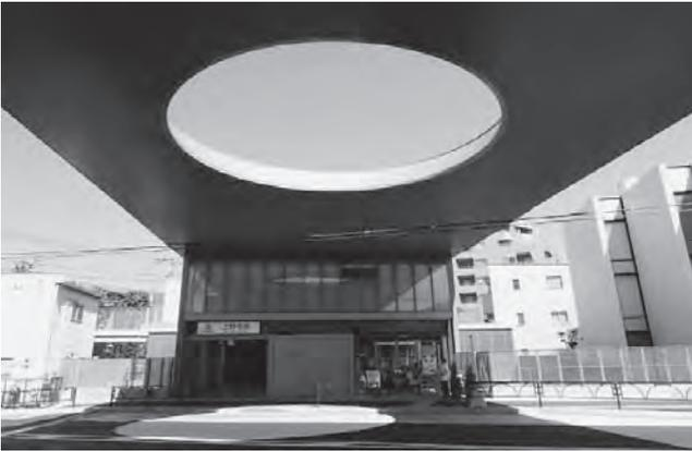
Fig. 3 Circular opening of large roof looked up from the station plaza
