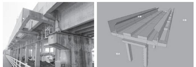
Fig.11 3D model of a snow damage countermeasure structure.
